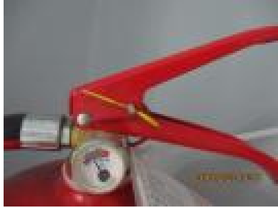
Pressure gauge of fire extinguisher.JPG
