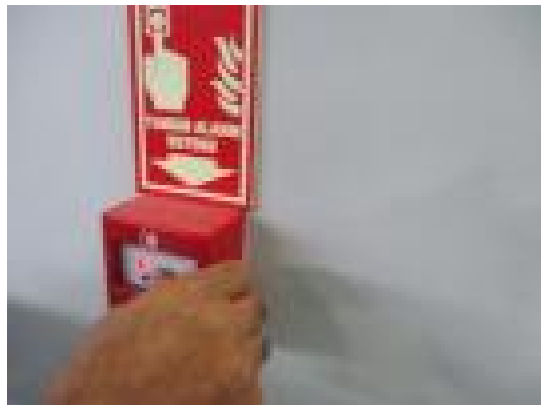
Testing fire alarm.JPG
